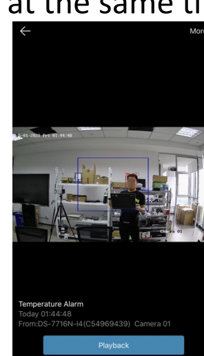
Alarms in App
